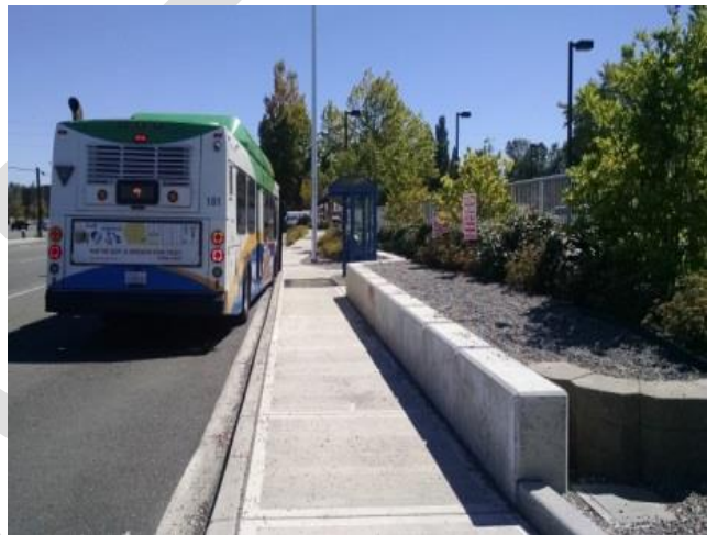
Post-construction facing east
