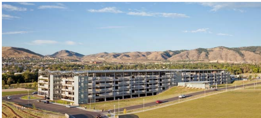
National Renewable Energy Laboratory (NREL) Garage in Golden, CO
