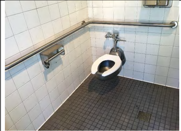
Toilet in public restroom
