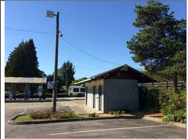
Phone line to the Utility Building
