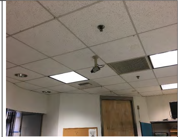
Ceilings and walls
