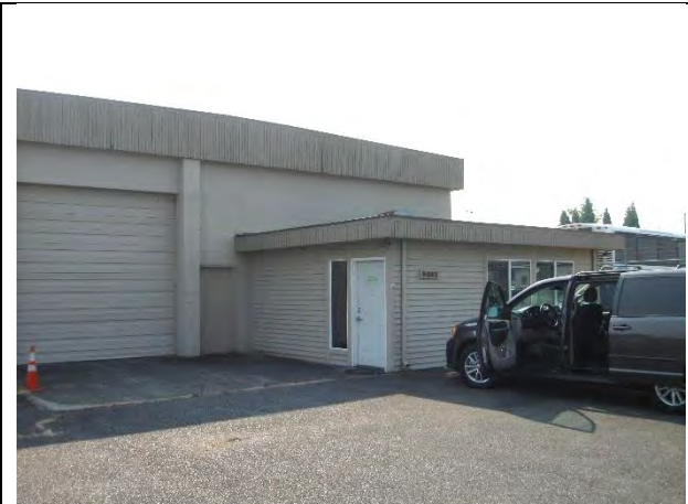
Office space add-on on west side
