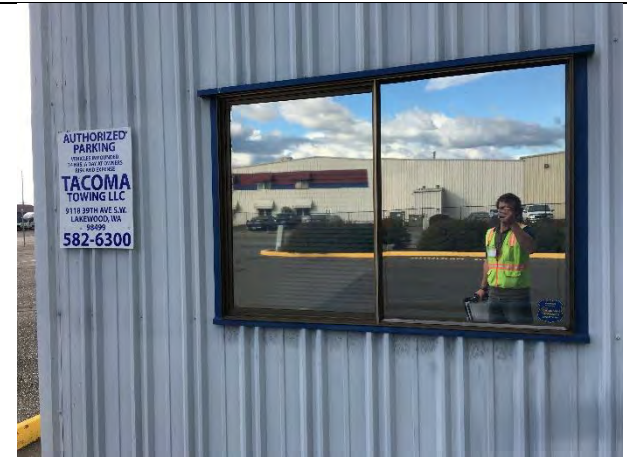
Exterior windows, east wall
