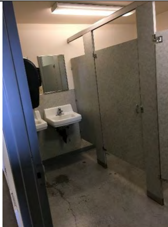
Men's restroom partitions
