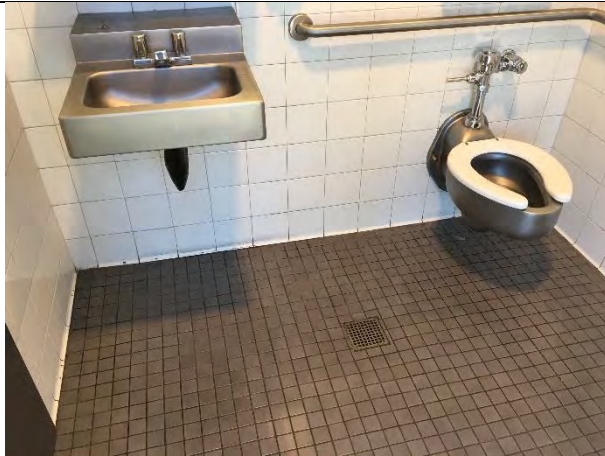
Public restroom wall and floor
