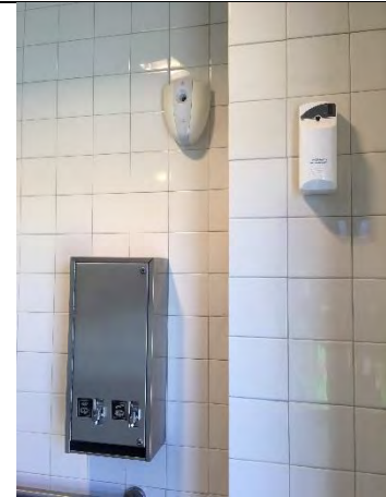
Driver restroom wall-hung accessories
