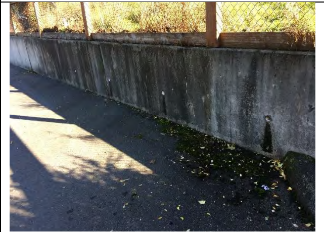
Retaining wall with relief drains
