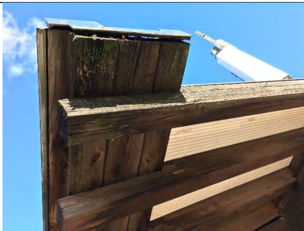
Utility building view under gutters
