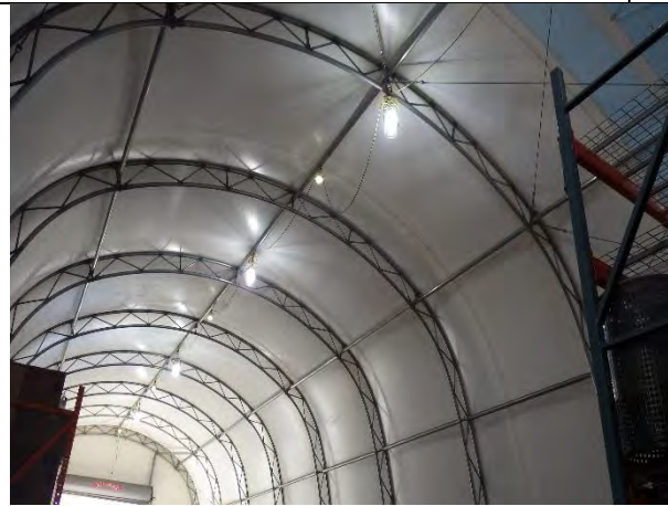
Festoon lighting modified to supply power to larger LED luminaires
