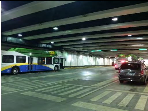
Underground retaining walls
