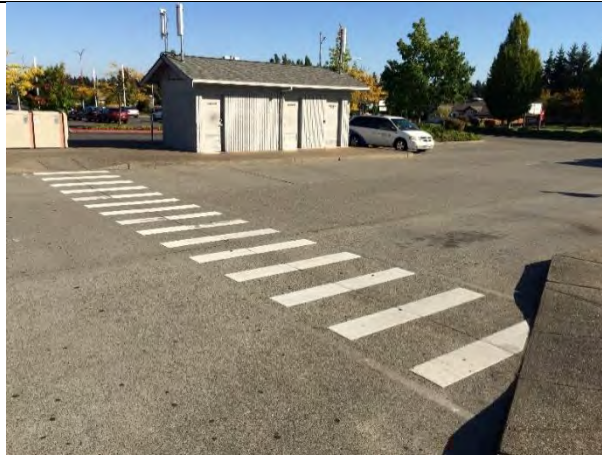
Pedestrian crosswalk paint in adequate condition
