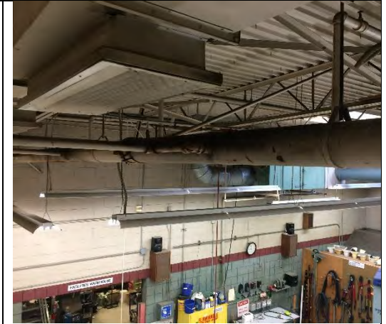
Interior of shop, looking northeast
