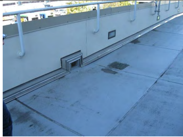
Roof has good slope and appears to be draining properly
