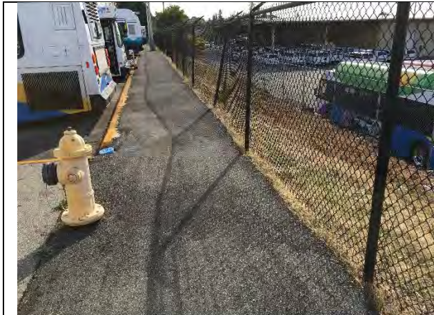
Vertical fence posts are bowed out and the top rail has been bent.
