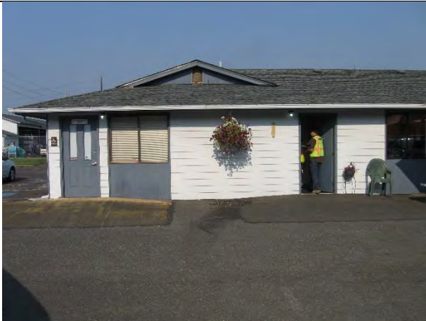
East wall entry of service supervisors building
