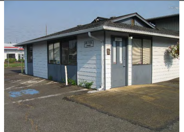
South wall of service supervisors building
