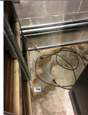
Storage room adjacent to the facilities maintenance work room
