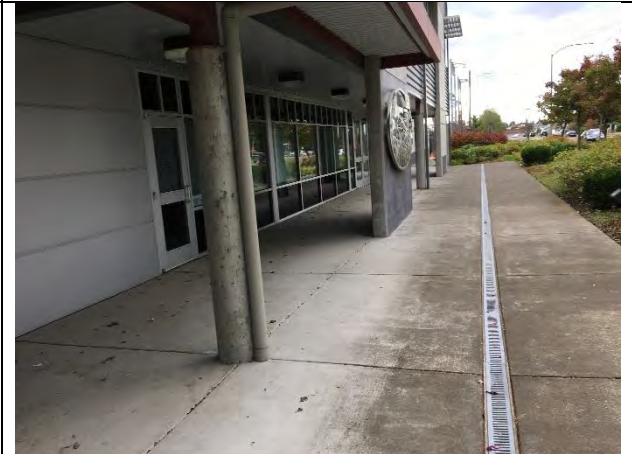
Concrete columns and canopy at north side of building
