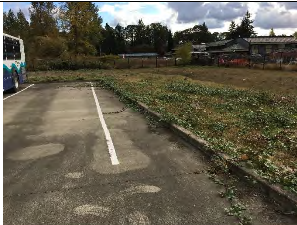
Vegetation overgrowth at southwest corner of parking lot
