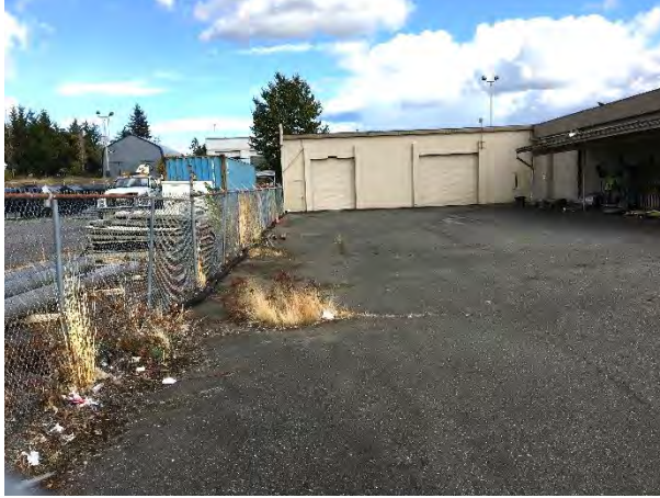
Weeds growing up against the fence
