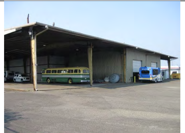
Southeast corner of the metal building
