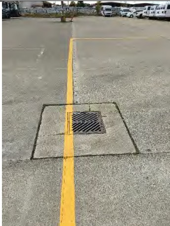
Storm drain in parking area
