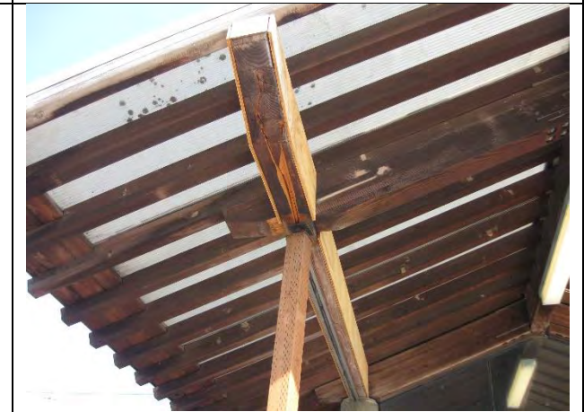
North bus shelter with wood post shoring roof beam
