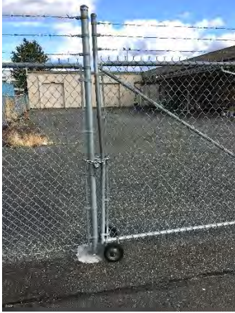
Rolling entrance gate on west side of property
