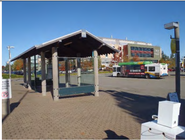
West bus shelter
