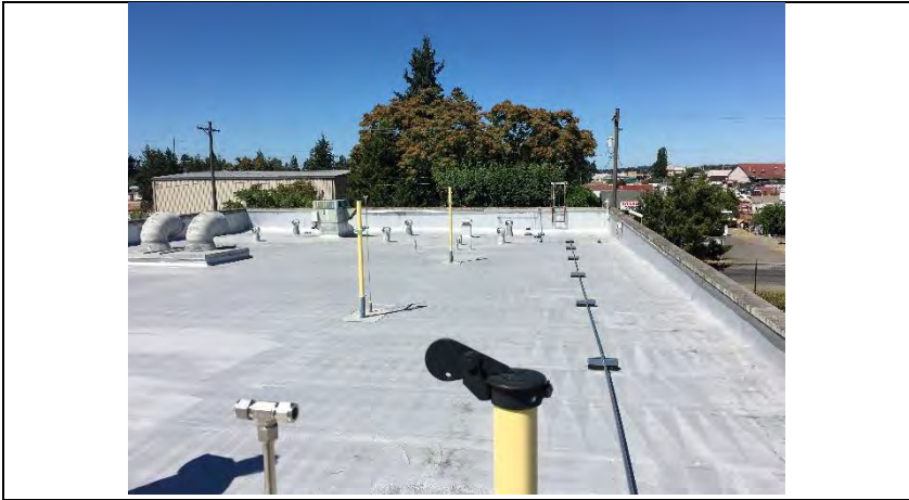
Roof appears to be properly sloped and drainage is functioning properly
