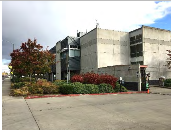
View of northwest corner of building and west entry gate
