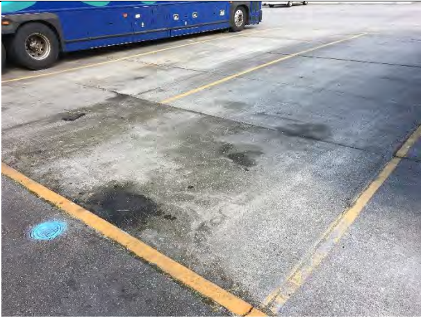
Low spot in concrete and sidewalk on southwest side of building that has settled
