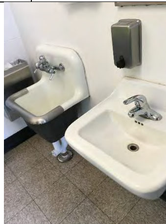
Sink and slop sink in driver restroom facility
