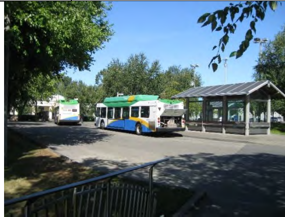
Concrete panels are in adequate condition
