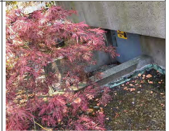
The personnel access to the fan room is limited to a door approximately 3'x3' that is located in a vault on the north side of the room
