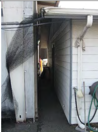
North wall of service supervisors building and narrow gap to metal building
