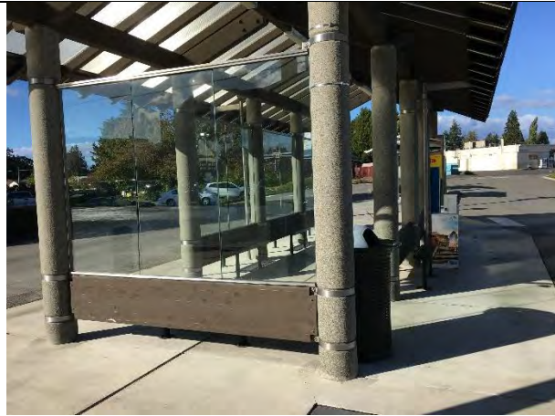
Glass in large shelter
