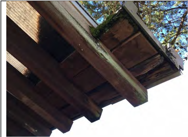
Utility building eaves
