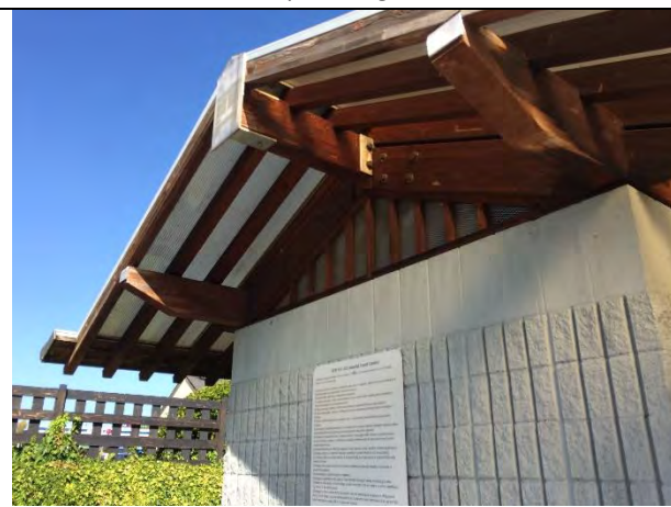
Utility building eave
