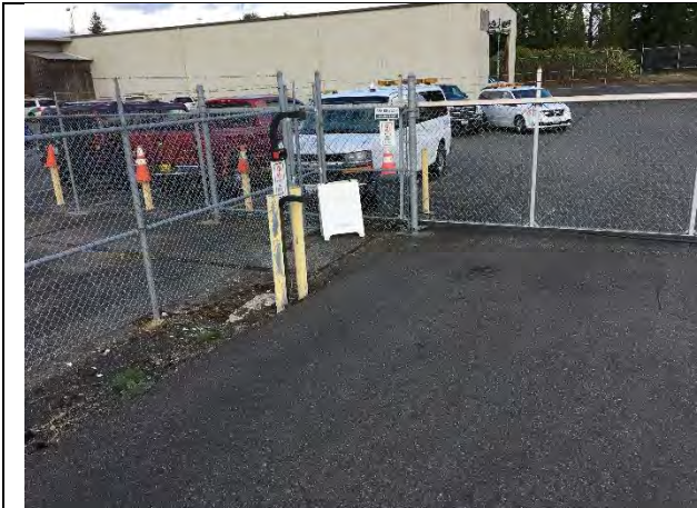
Electric entry gate on southwest corner of property
