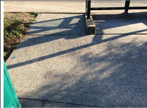
Bus shelter concrete in good condition
