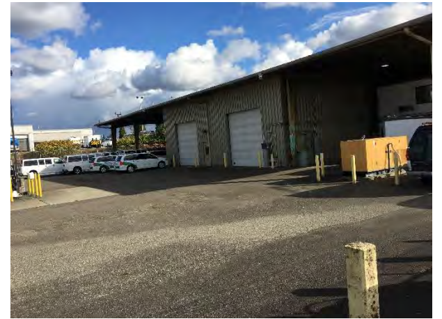
Bollards in front of generator and garage doors
