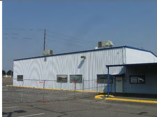
South side of building
