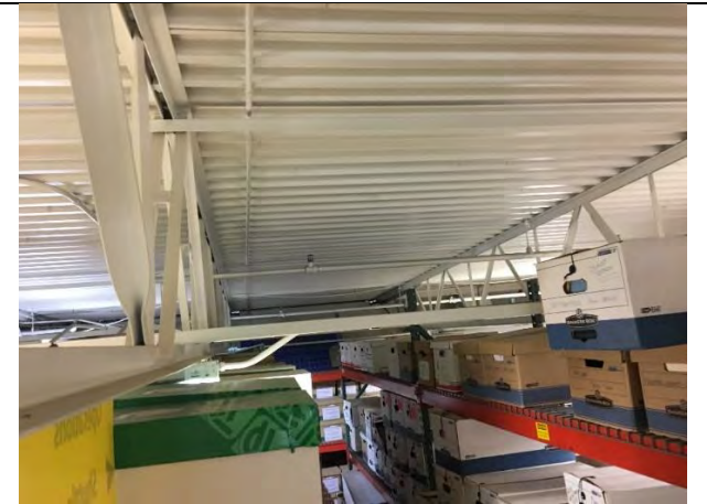
Rack storage in mezzanine
