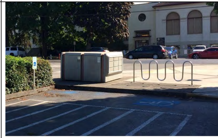
Bike Locker and Bike Rack are in good condition
