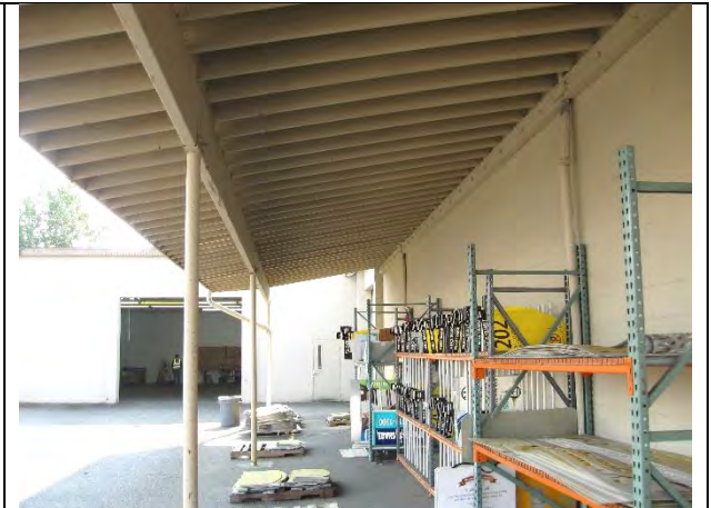
Warehouse exterior under shed roof on north side
