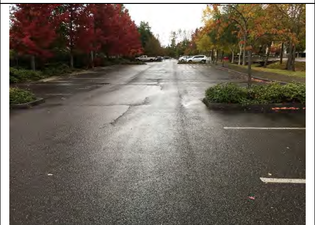
Asphalt in parking area
