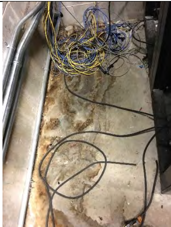
Storage room adjacent to the facilities maintenance work room
