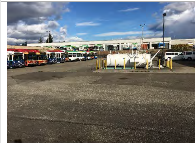
Bollards around fuel tank
