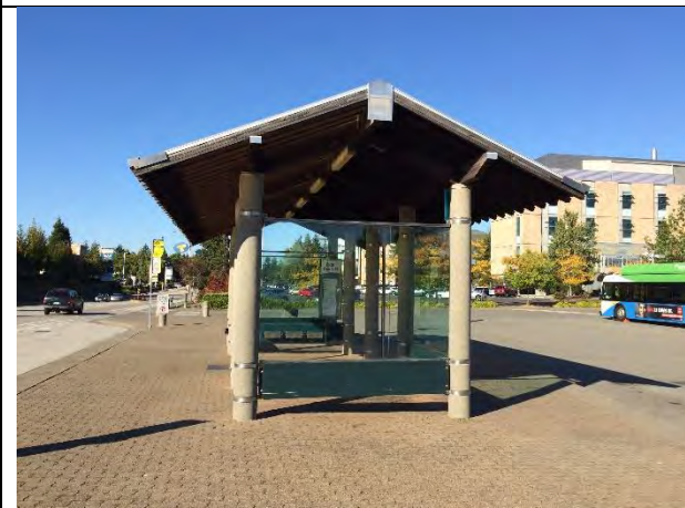
West bus shelter
