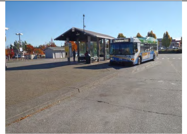
East bus shelter with utility building in background
