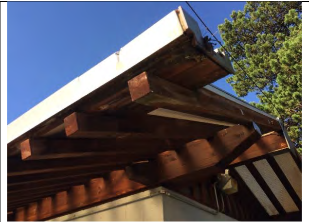
Utility building rafters
