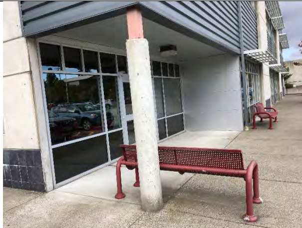
Southwest corner of building
