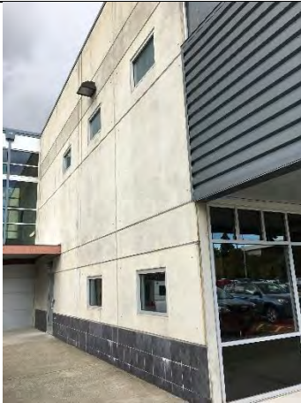
Southwest corner of building
