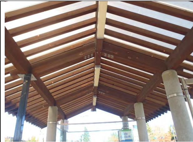
Bus shelter framing and roofing
