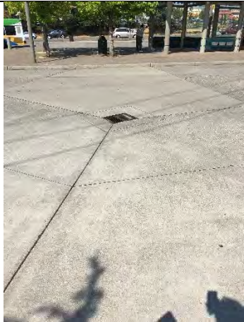
Storm water grate in bus driveway
