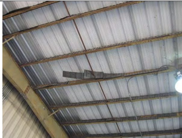
Underside of roof at the metal building on the west end
