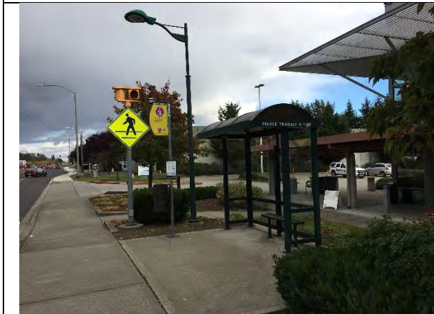
Bus shelter at front entrance
