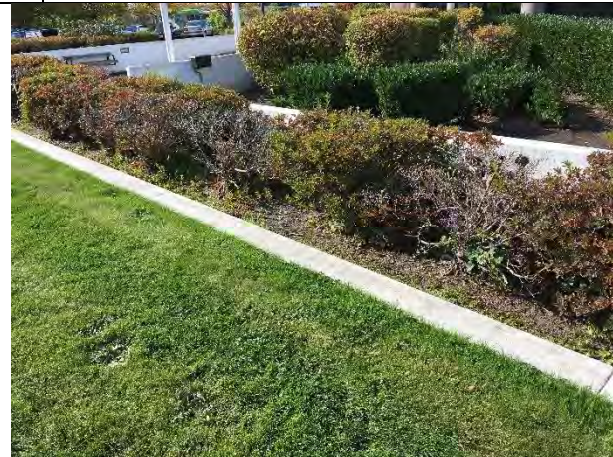
Landscaping is dying in several areas around building including by the front sign, on both sides of the vehicle entrance/exit gate, and by the backup generator
