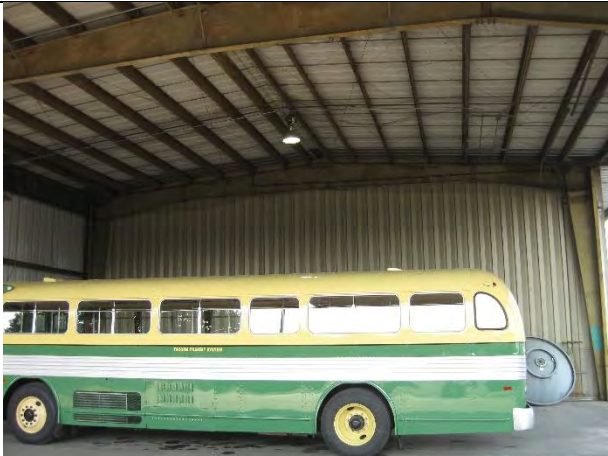
East wall of radio maintenance area, vintage bus parking
