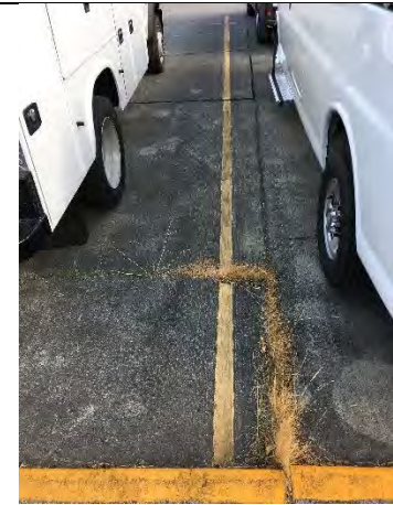
Cracks in panels on the southwest side of the building
