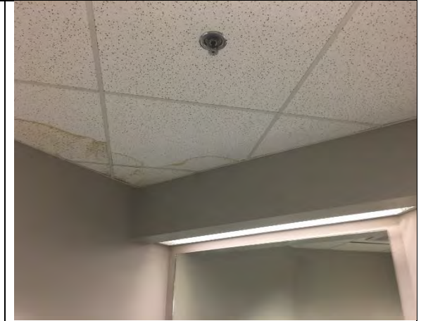
Bus Shop ceiling
