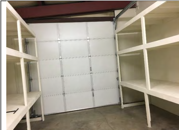
Rollup garage door from interior
