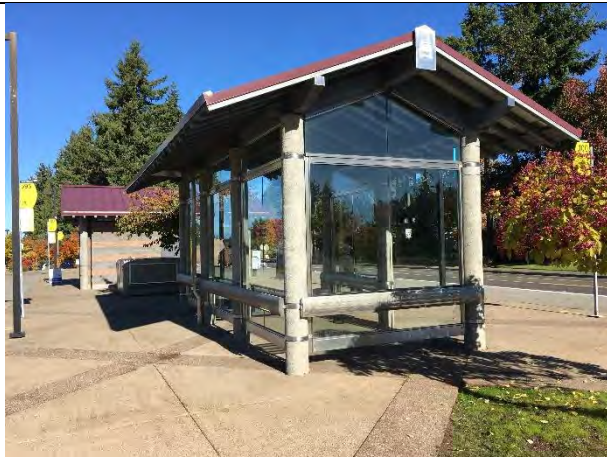
South bus shelter
