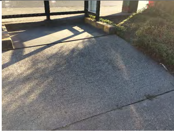
Bus shelter concrete in good condition
