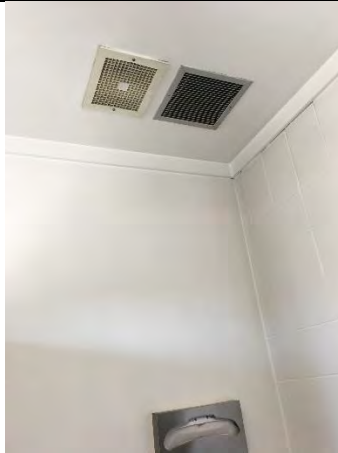
Exhaust fans in restrooms
