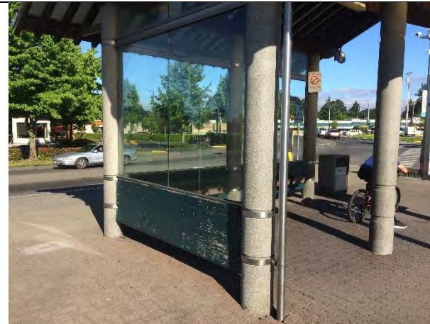
Bus shelter glass and wooden side panels
