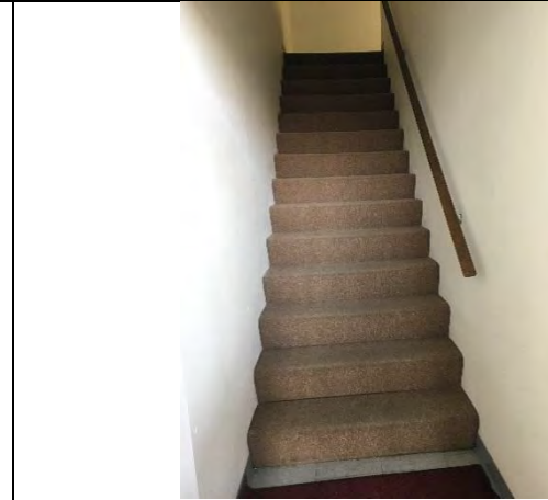
Stairs to second level in two story office at the west end of the metal building.
