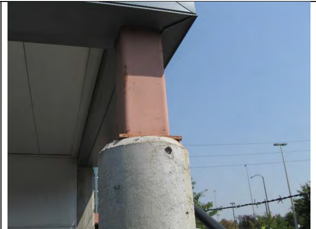
Steel beams and concrete column
