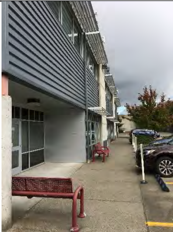
South wall of building
