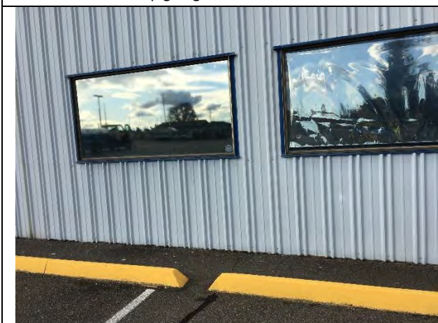
Exterior windows, south wall
