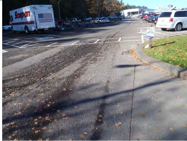
Looking West into Metro Parks parking area
