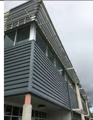
Southwest corner of building showing upper metal siding and sun screens
