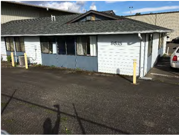
Bollards protecting building and equipment
