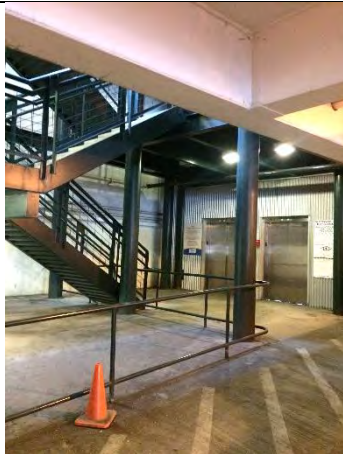
Elevators and stair case
