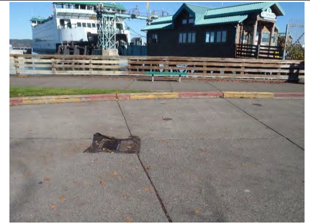
Storm drains on site appear adequate
