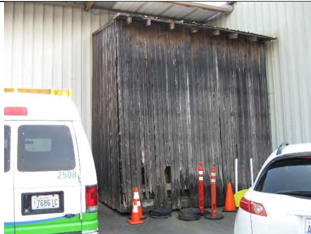
Wood frame shed at "L" corner
