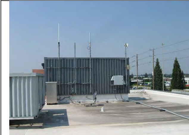
Roof looking north at penthouse, showing antenna structures
