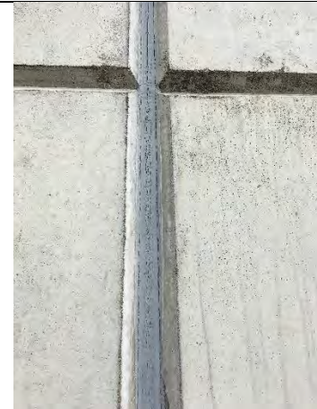
West wall of building showing caulk joint between precast concrete panels
