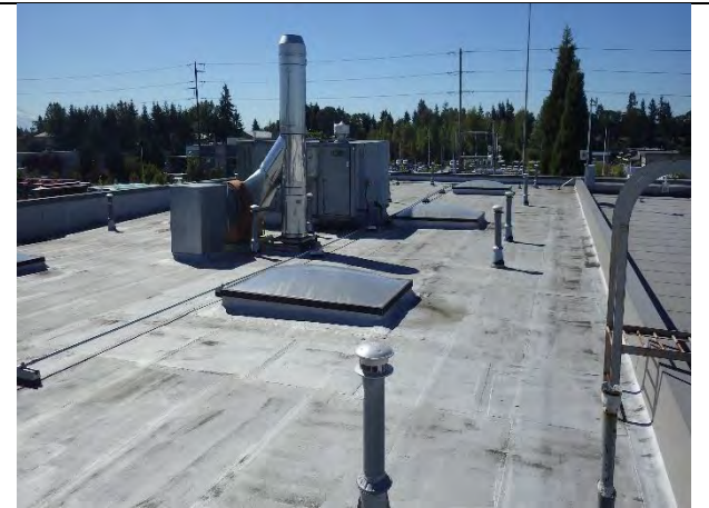
Roof and skylights
