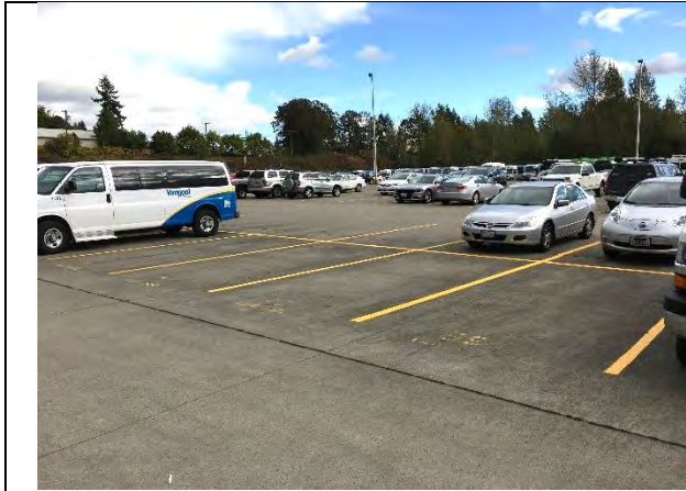
Painted numbers on parking stalls fading
