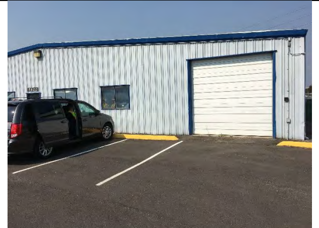
Roll up garage door at east wall
