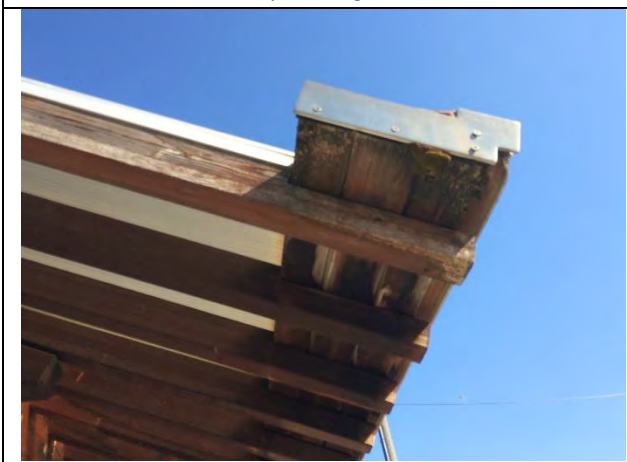
Utility building eave
