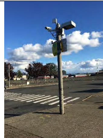
Cameras installed around site
