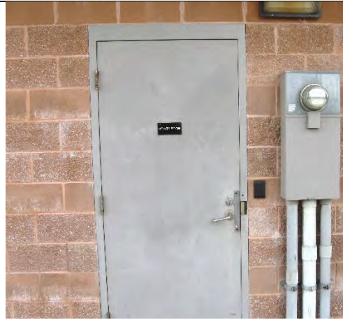
Utility room door
