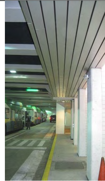
Slatted Ceiling in Tunnel
