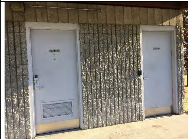
Utility building doors
