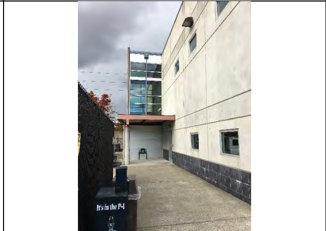
Downspout from roof at west side of building
