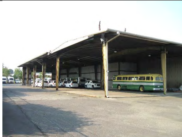
East wall of metal building, showing south wing of "L"
