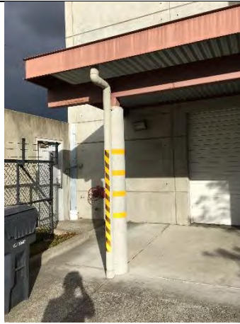
Canopy at shipping dock, northwest corner
