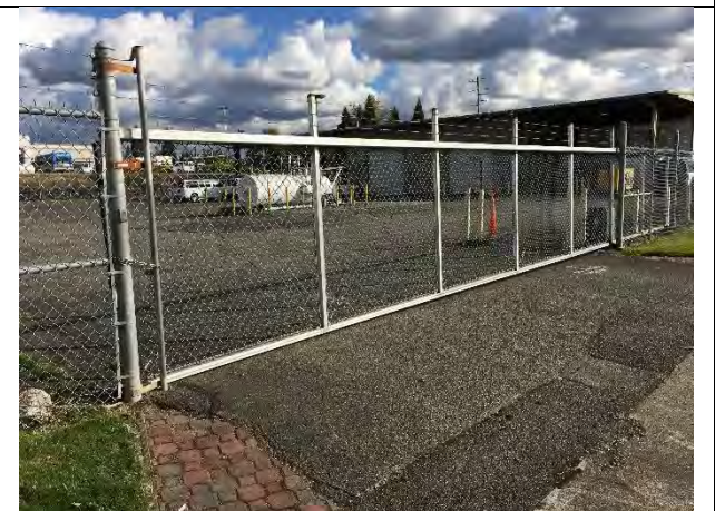
Chained manual gate on northwest corner of property
