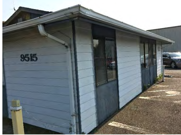
Southwest corner of service supervisors building
