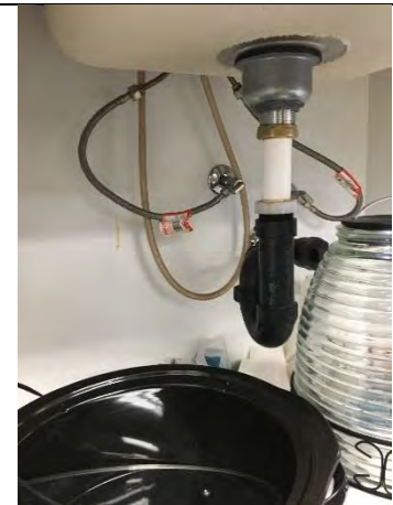
Service supervisor building kitchen sink in common area
