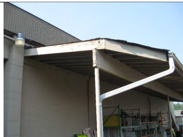
Exterior gutters and downspouts
