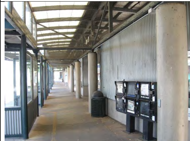
Pedestrian walkway concrete in good condition
