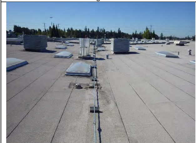
Roof and skylights
