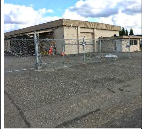
West side of building and warehouse, site asphalt and fence
