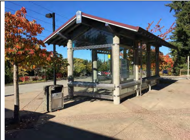
North bus shelter
