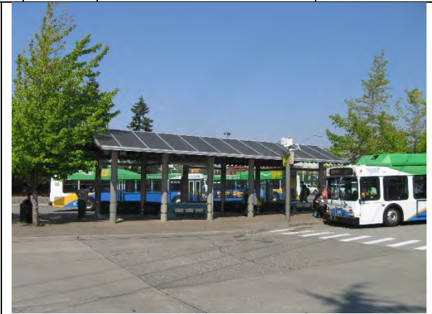
South bus shelter structure is in good condition
