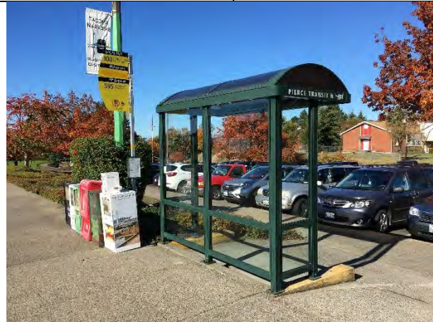
Bus Shelter on 6 th Avenue
