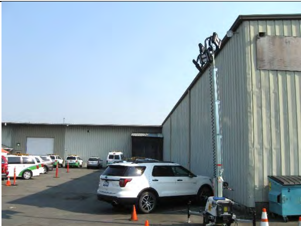
Southwest corner of "L", south wall of radio maintenance area
