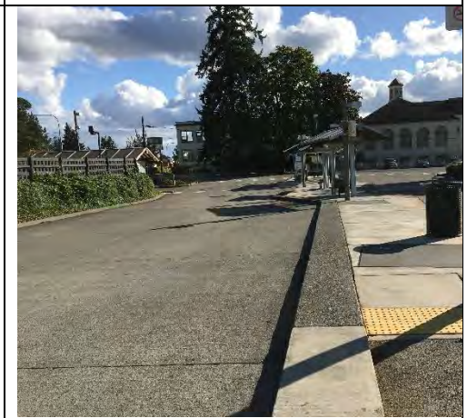
Passenger walkways and waiting areas
