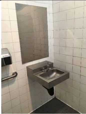
Sink and mirror in public restroom
