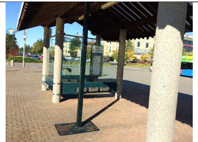
West bus shelter with middle column replaced with steel post
