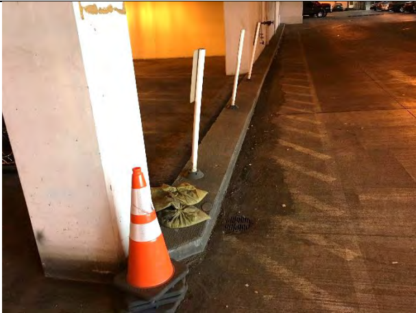
Water drainage in the west parking structure
