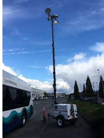
Temporary lighting set up all around site
