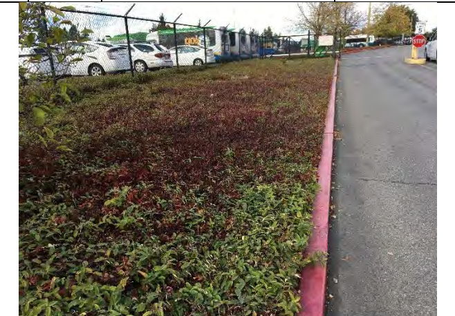
Landscaping is dying in several areas around building including by the front sign, on both sides of the vehicle entrance/exit gate, and by the backup generator
