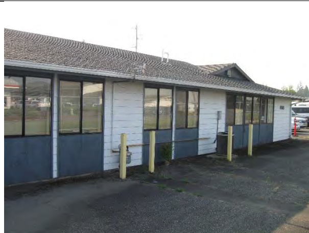
West wall of service supervisors building
