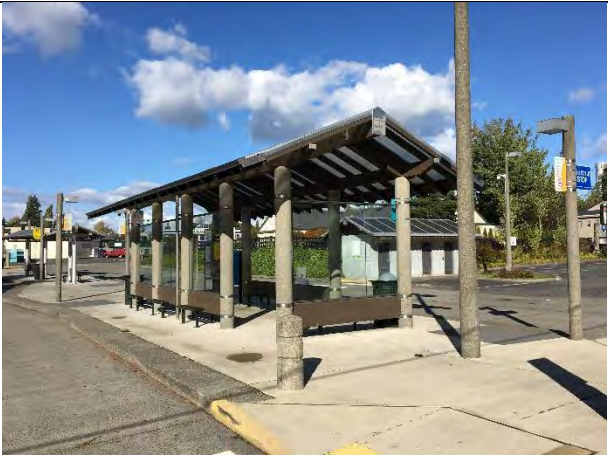
Large bus shelter
