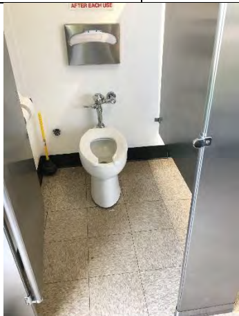
Toilet in driver restroom facility
