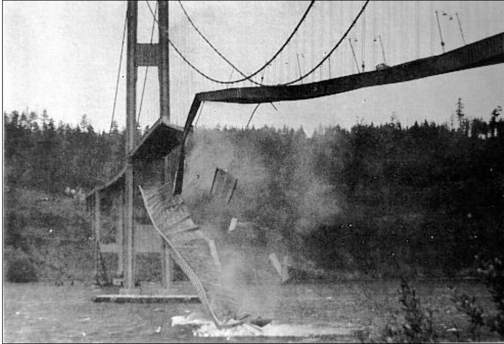
Figure 4.9-5 Tacoma Narrows Bridge – November 7, 1940 Windstorm
