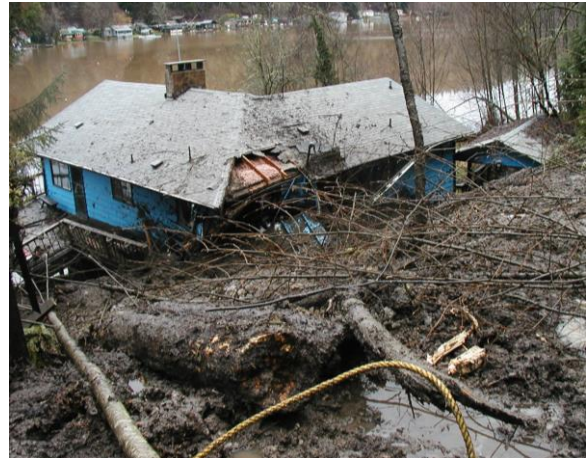
Figure 4.3-4 Ski Park Road – Landslide 01/31/03
