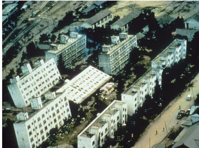
Figure 4.2-4 Liquefaction, Niigata Japan 1964
