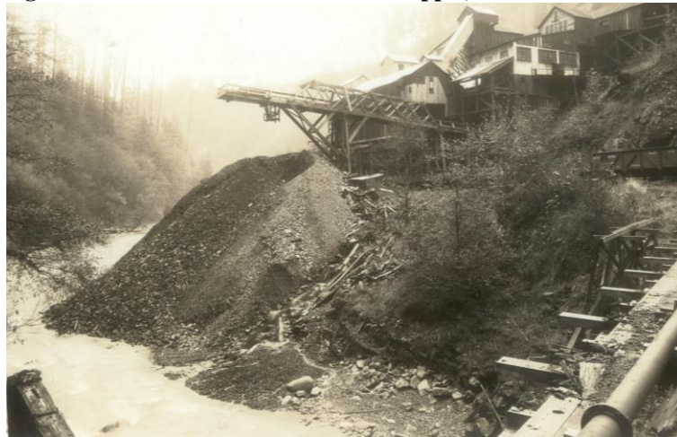
Figure 4.11-3 Pacific Coast Coal Mine Tipple, Carbonado 220
