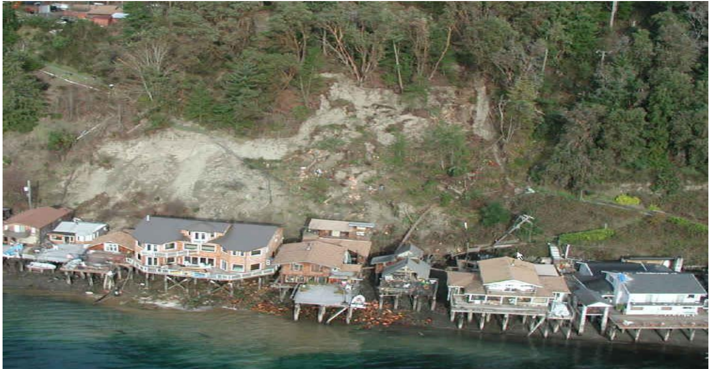
Figure 4.2-3 Salmon Beach, Tacoma Washington – Following Feb. 2001 Earthquake
