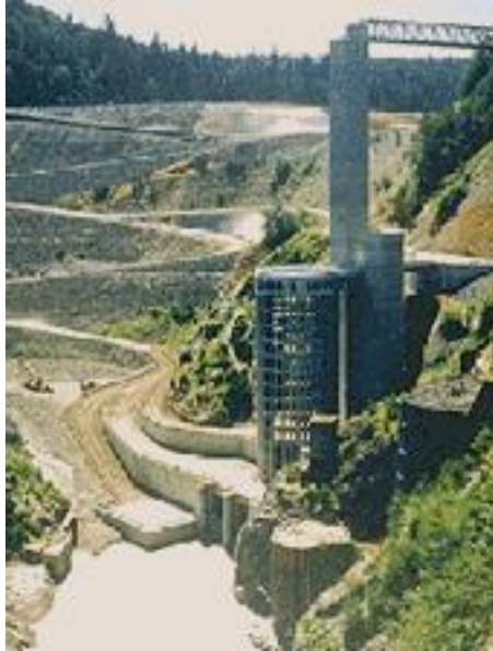
Figure 4.15-2 Mud Mt. Dam Intake 273
