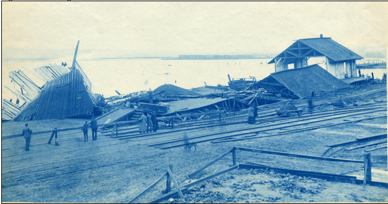
Figure 4.4-6 Damage in Tacoma from the 1894 Tsunami 77
