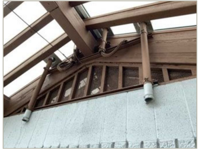
2 - WAITING STATION - ROOF STRUCTURE
