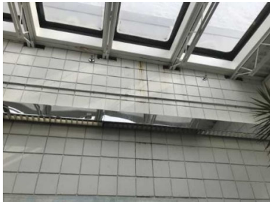
Water leaks occurring around the lobby skylight. - AssetCALC ID: 3441469
