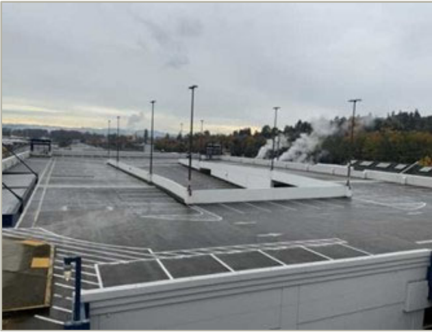
1 - ROOFTOP LEVEL OF GARAGE
