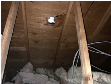
Hole in roof. - AssetCALC ID: 3345106
