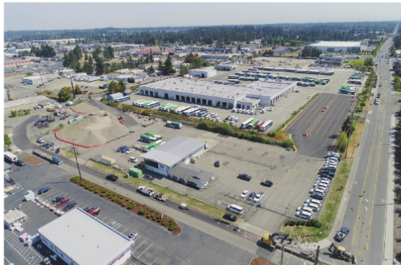
An aerial view looking east of the Pierce Transit Maintenance & Operations Base Improvement (MOBI) project site.
