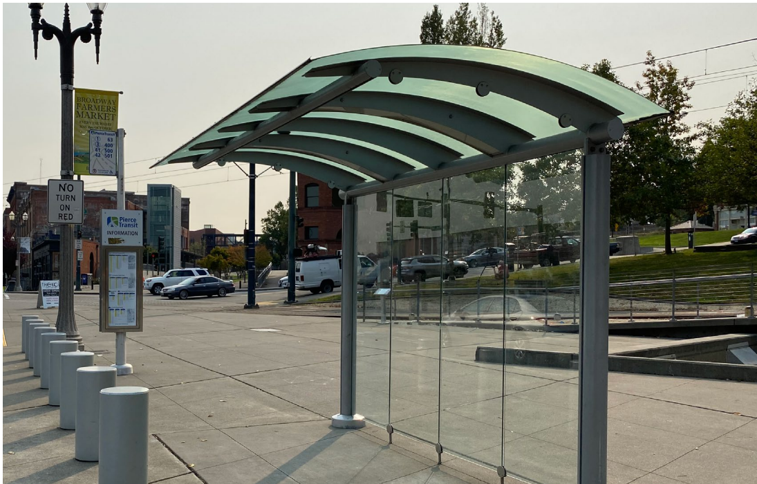
Custom shelter example (found at Tollesfson Plaza)
