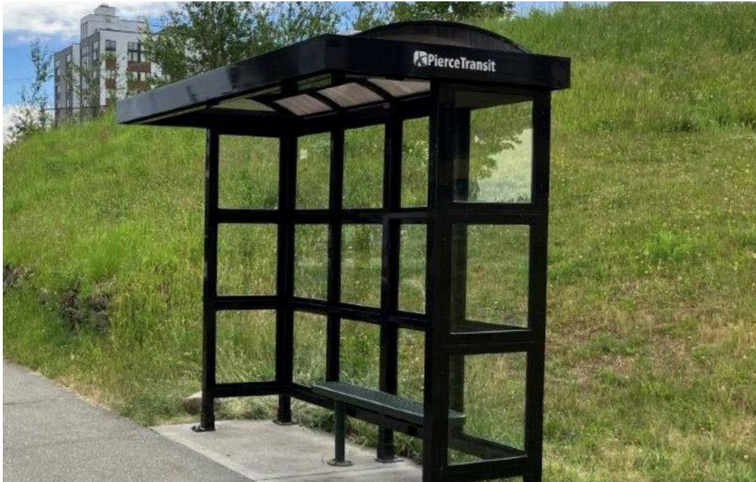
Cantilever Shelter (Pierce Transit's current standard)
