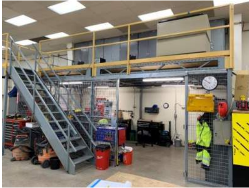
Prefab mezzanine along north wall.
