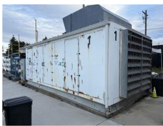
Site slope is evident at base of large units
