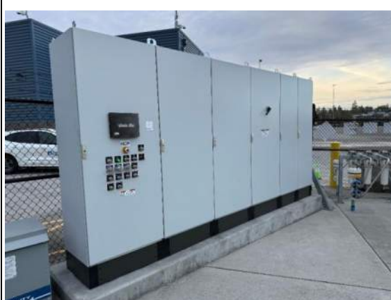
Site slope is evident at base of large panel
