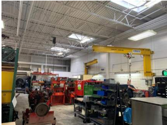
Jib cranes in engine shop
